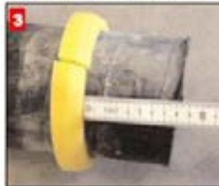
Positioning of the weld-on ring
